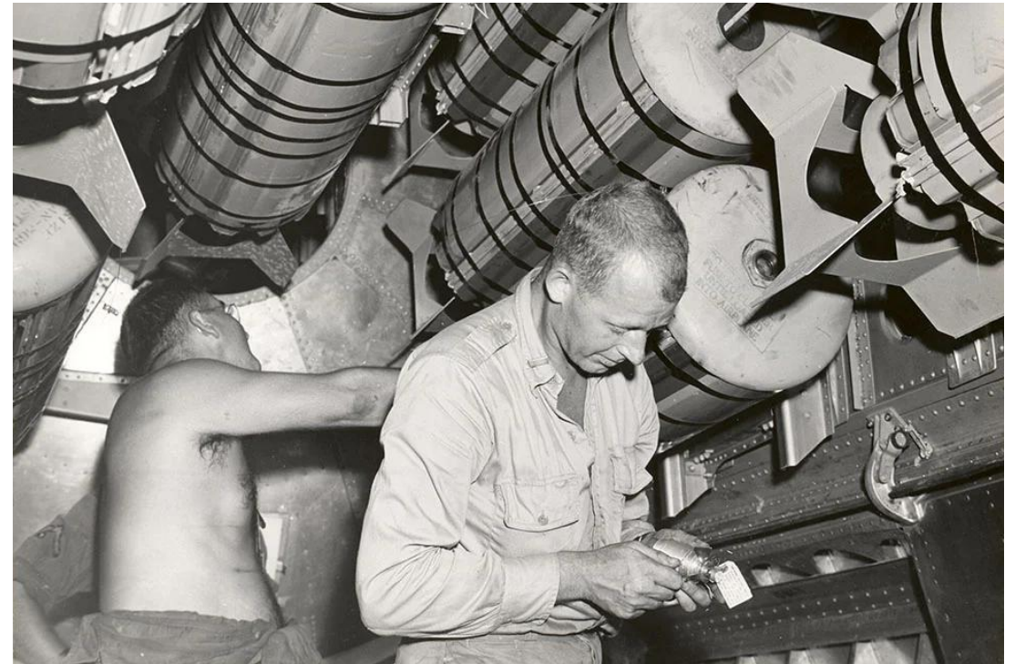
Armorers fuse 500lb incendiary clusters that have been loaded into a 500th Bomb Group B-29 Superfortress. (National Archives)
