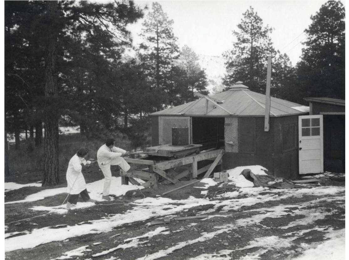
Remote handling of a kilocurie source of radiolanthanum for a RaLa Experiment at Los Alamos
