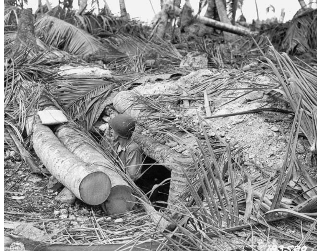
After its original occupants have been killed, an American soldier stands in the entrance to a Japanese bunker on Butaritari. Heavy coconut logs were used to reinforce the enemy strongpoint.
