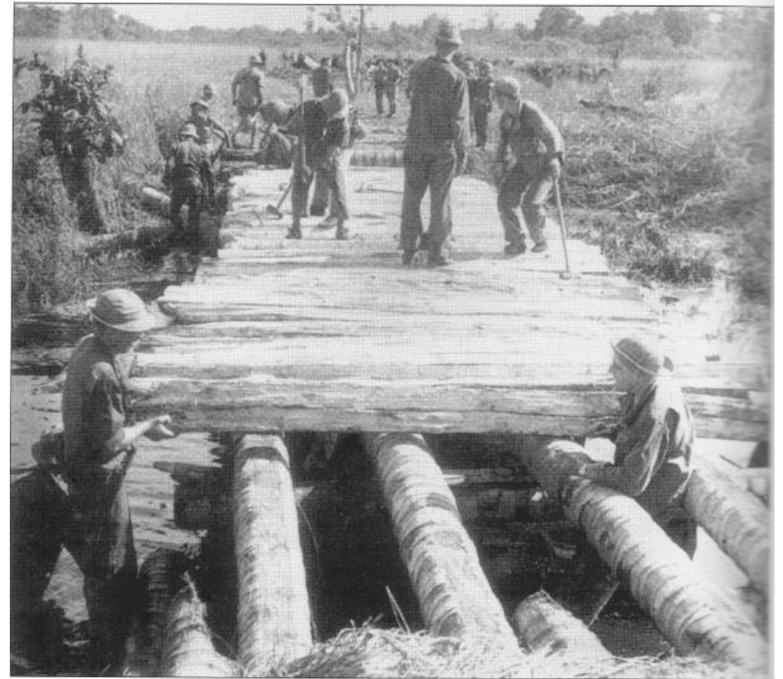
American engineers strengthen the bridge over Simemi Creek, ready for the Stuarts to cross for the attack. (US Army)
