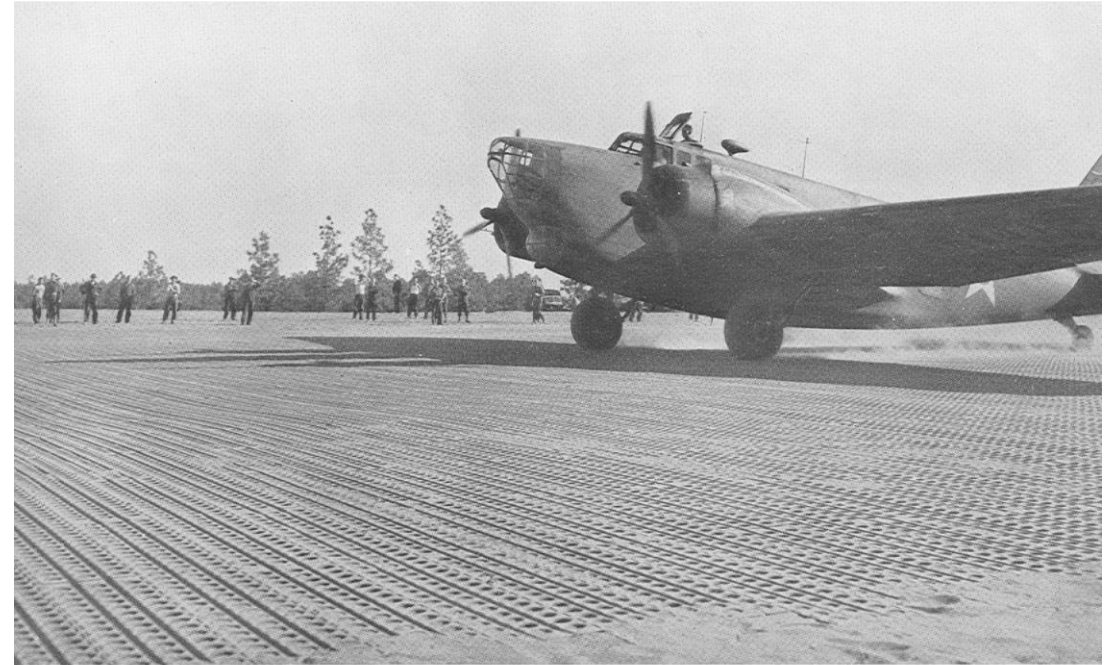
FIRST TEST LANDING ON STEEL MATTING, CAROLINA MANEUVERS, 1941
