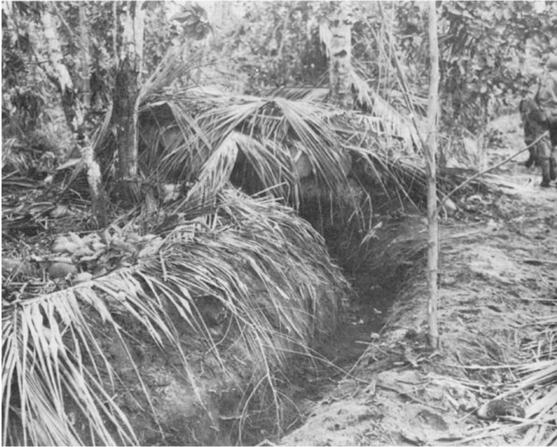
COCONUT LOG BUNKER WITH FIRE TRENCH ENTRANCE in the Buna Village area.
