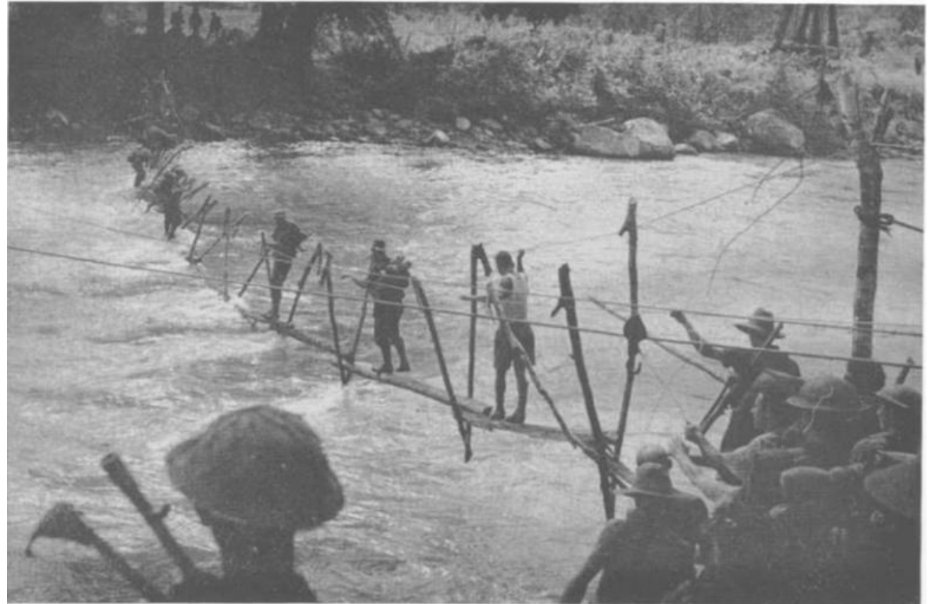
(Australian War Memorial) Crossing the Kumusi River at Wairopi on a makeshift bridge constructed by Australian engineers. November 1942.
