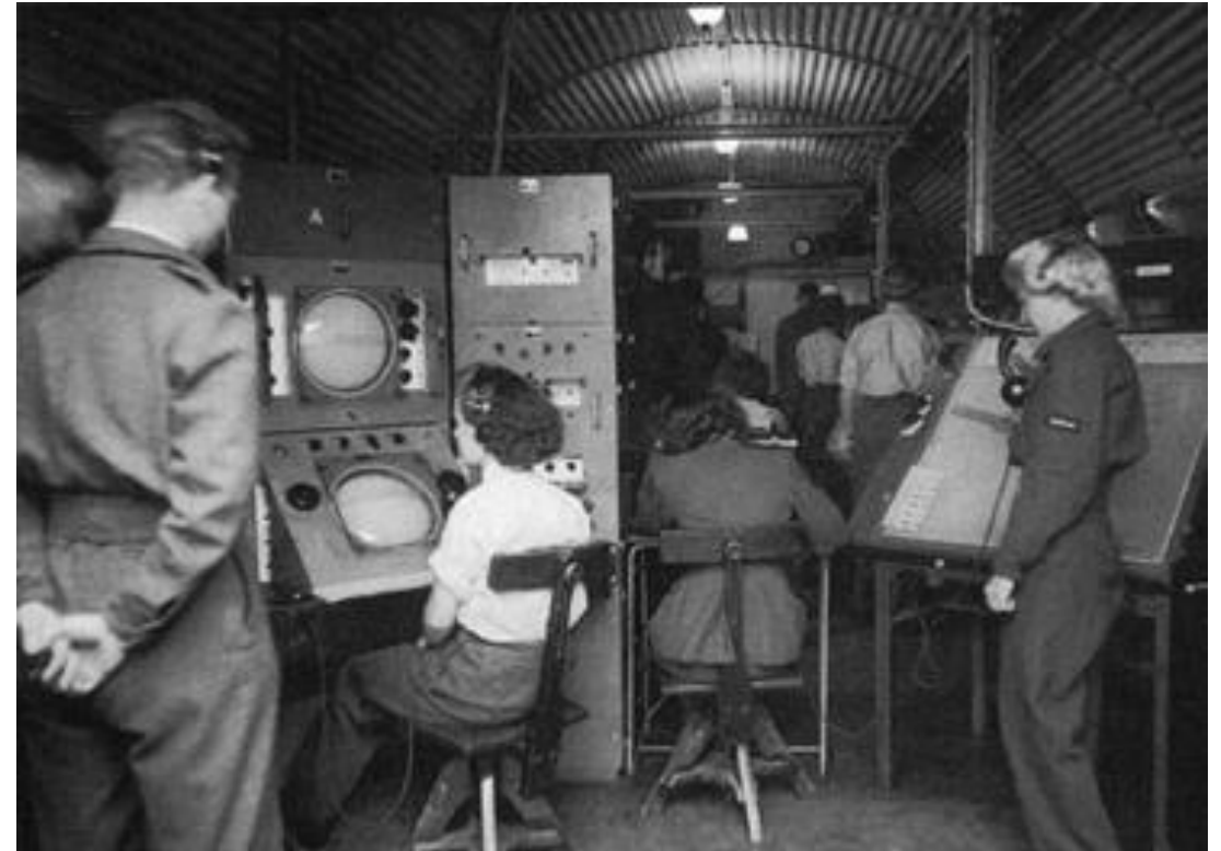
The left side of this image shows an Oboe navigation console. The two CRTs, some of the largest built during that era, were used for gross and fine distance measurement.
