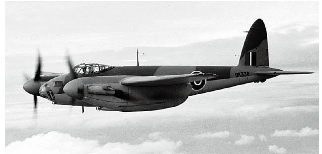
192 squadron Mosquito with aerial for Mandrel radar jammer.
