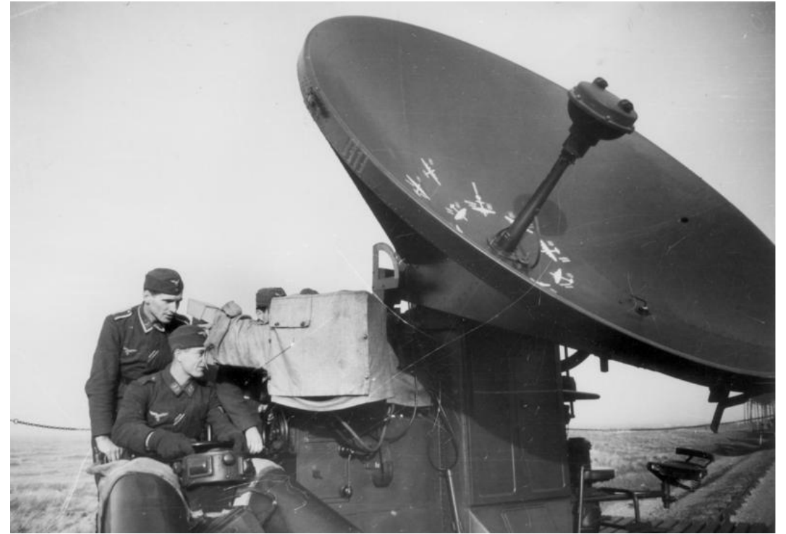
Würzburg D in use. The quirl conical scanning antenna is prominent.
