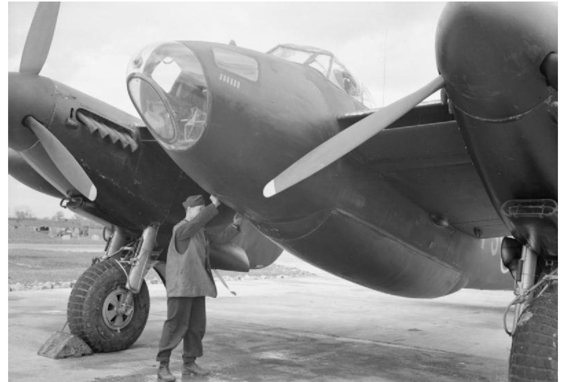
A De Havilland Mosquito B Mark IV (modified) of No. 692 Squadron RAF of the Light Night Striking Force, at Graveley, Huntingdonshire, showing the enlarged bomb-bay, fitted to accommodate the 4,000-lb HC bomb.
