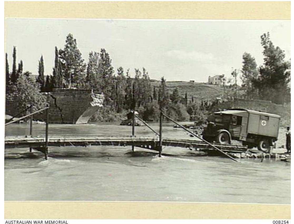
AUSTRALIAN AMBULANCE CROSSING BRIDGE CONSTRUCTED ACROSS THE LATANI RIVER BY AN ENGINEERS UNIT TO REPLACE BRIDGE BLOWN UP BY THE RETREATING FRENCH. (NEGATIVE BY F. HURLEY).
